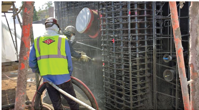
Figure 10 – 10-1: Illustration of shotcrete application method. 10-2: Three-dimensional color simulation indicating deflection and acceleration of formwork. 10-3: Two-dimensional color simulation indicating deflection and acceleration of formwork. 10-4: Stand-alone mock-up during shotcrete application.
